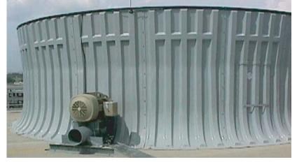
Dynamic Fabricators high quality fiberglass reinforced polyester fan stacks are manufactured in our ISO 9002 Certified Manufacturing Plant. Our stacks have an engineered laminate schedule manufactured to precise standards ensuring consistency and excellent quality. Each stack has a belled inlet and conical, diverging exit for reduced air pressure drop losses and
